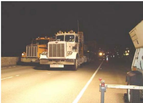
The I-90 load test involved loading trucks and driving them across the bridge to simulate the weight of light rail vehicles
