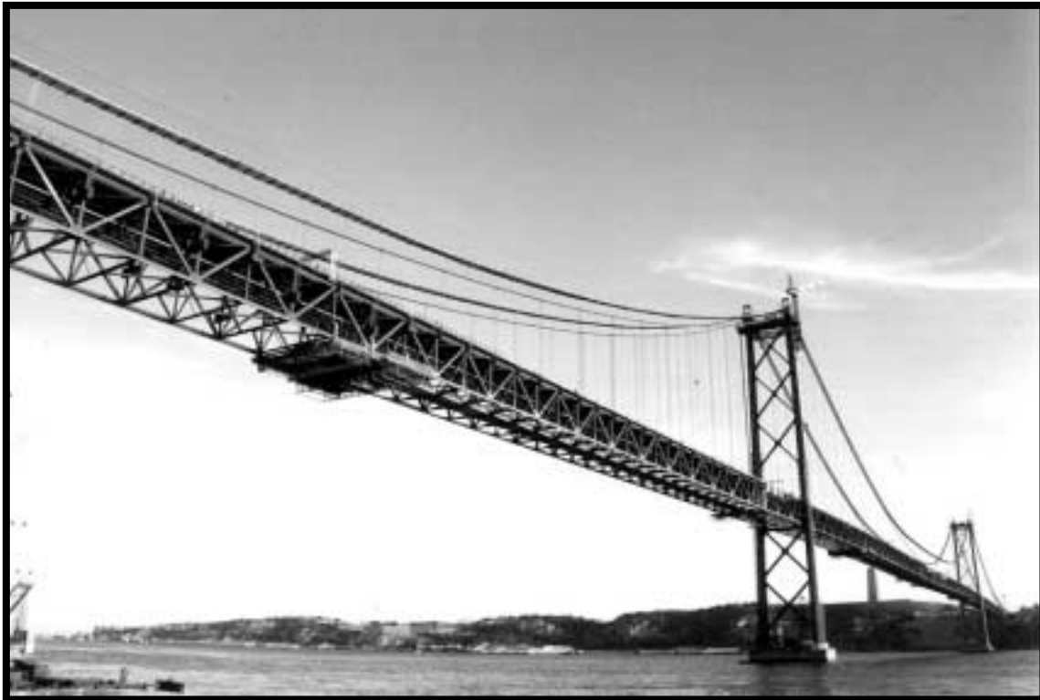
Photo #1 - Bridge Under Reconstruction
