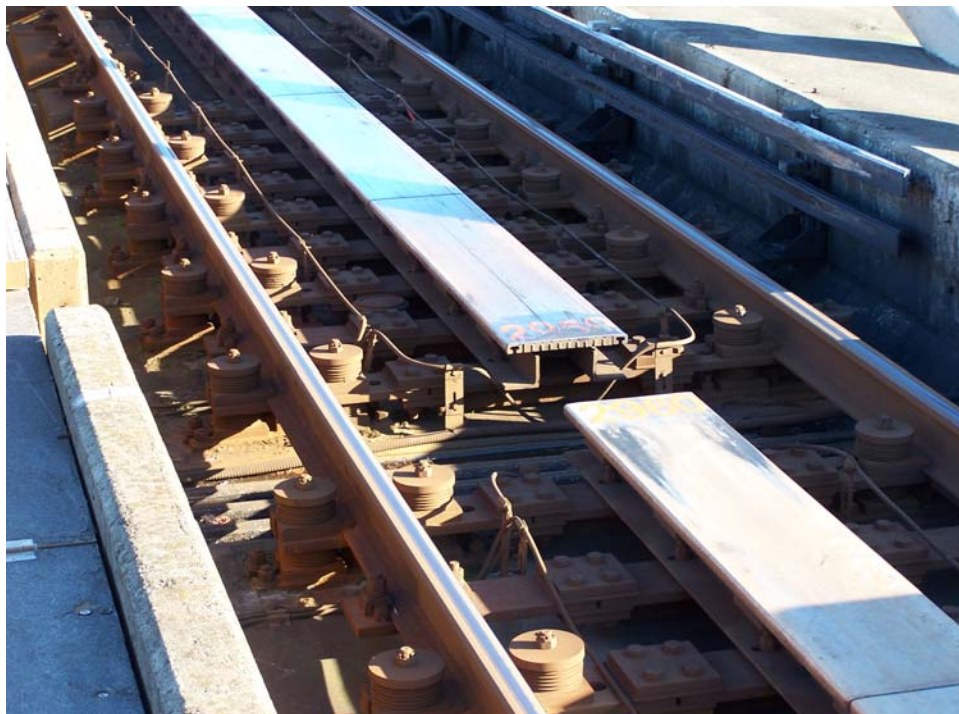
Photo 4: Close up of the bridge transition section
