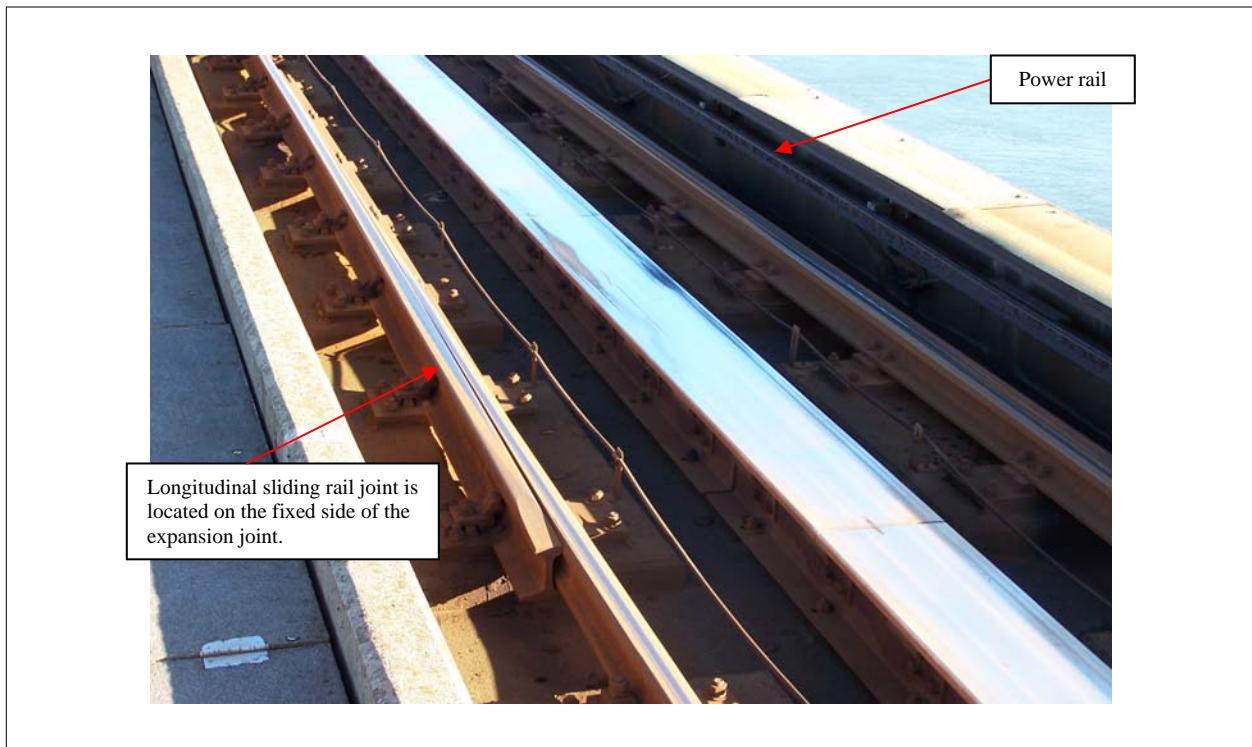
Figure 3. Fixed Side of the Rail Expansion Joint (matches to bottom of Figure 1)
