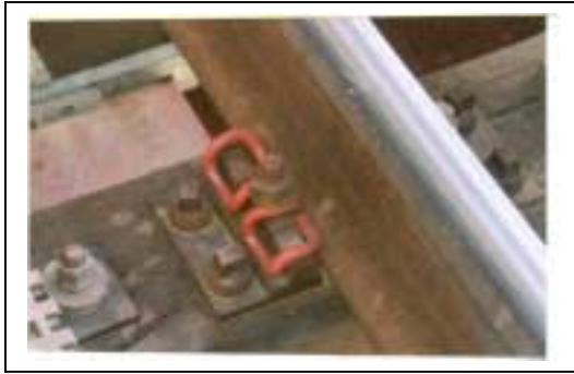
Photo #3 - Hook Bolt, Tension Clip and Clip Fixation
