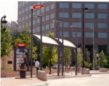
Metro Rapid station
