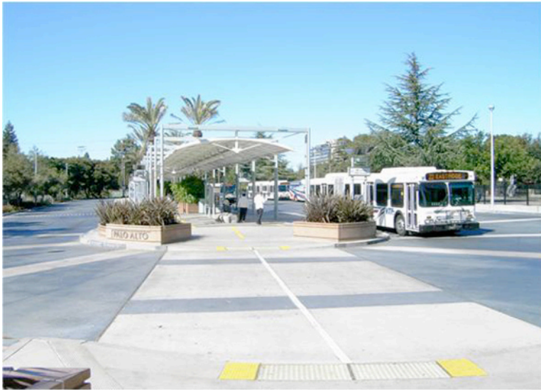
Figure 24 Palo Alto Transit Station
